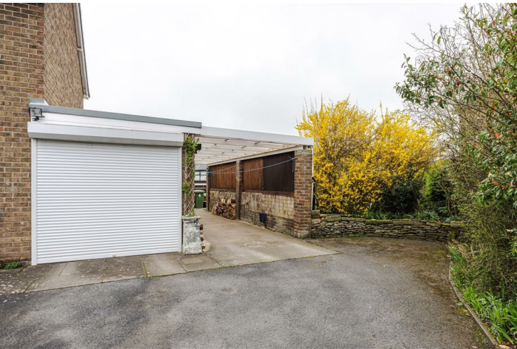
Garage 16'1" x 7'10" (4.92m x 2.39m)
